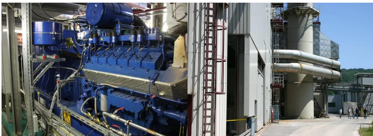
Figure 3-3: Combined heat and power unit and sludge incineration plant at WWTP Buchenhofen, Germany
