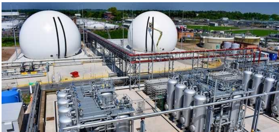
Figure 8-7: Minworth Sludge treatment plant. Showing the new THP plant in the foreground and the gas bags and MAD plant in the background
