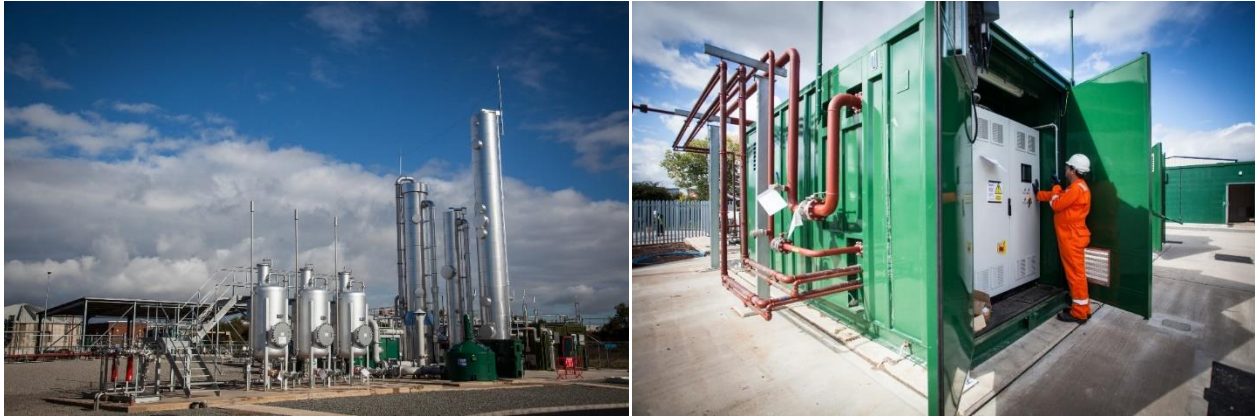
Figure 8-9: Biomethane Upgrading plant at Minworth (left) and Wartsila Gas compression unit (right)
